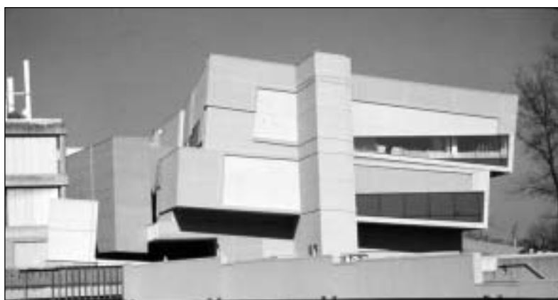
Aronoff Center for Design and Art, Peter Eisenman, 1996, University of Cincinnati, Cincinnati, Ohio.
